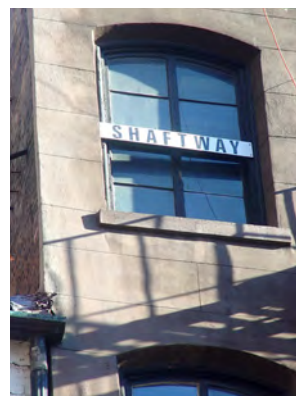
Figure 7.10. Exterior shaftway marking.
