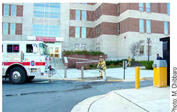
Figure 2.7. During initial operation at this structure, the first arriving engine crew is already using a fire lane, a fire hydrant, the fire department connection, and the key box. Interior operation will soon involve the alarm system, stairs, standpipe system, and other building features.
