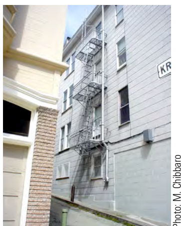
Figure 9.1. An exterior dry standpipe with an FDC on the bottom and a FHC at each fire escape platform.
