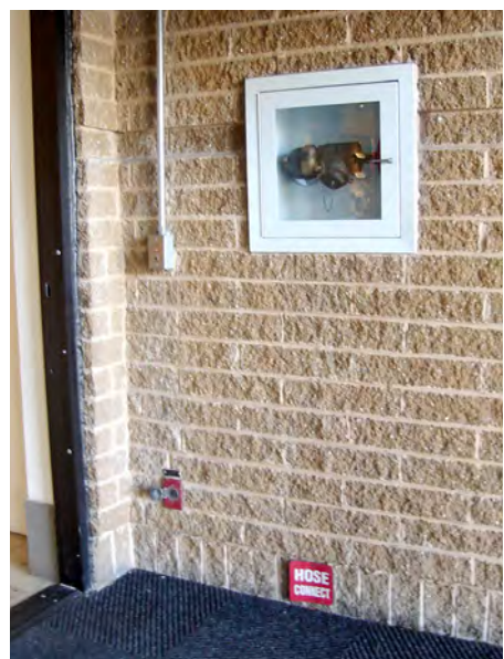
Figure 9.9. A remote FHC in a cabinet in a corridor. The sign near the floor is intended to help locate the cabinet in light smoke conditions. Note that the hose outlet is angled to facilitate connection of hose.
