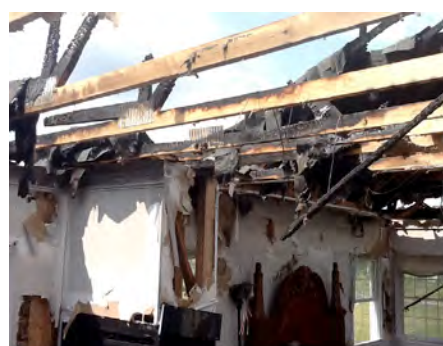
Figure 7.8. Wood trusses after an attic fire.
