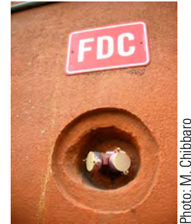
Figure 10.13. An FDC recessed into a wall. Note the notch on left prevents hose lines from kinking.
