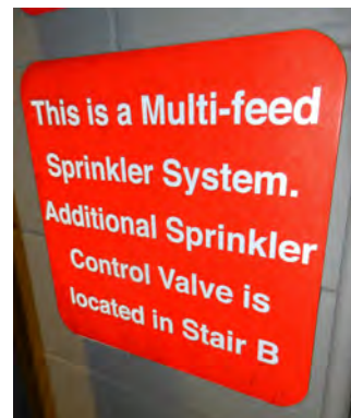
Figure 8.8. A sign near a sprinkler control valve indicating the location of the other valve that controls the same system.
